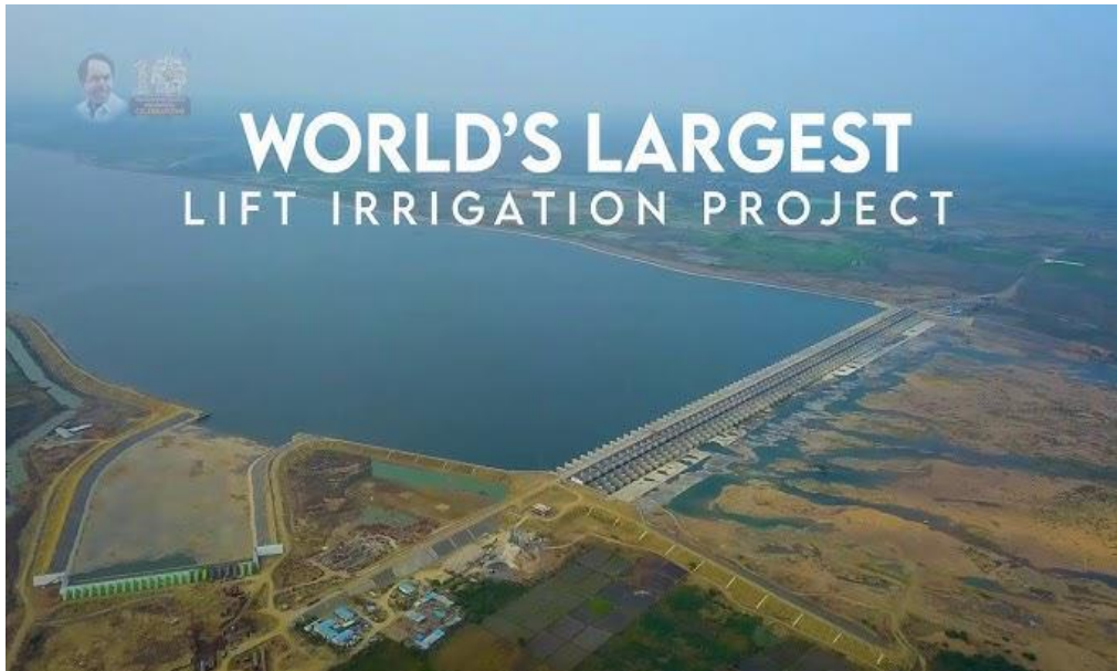
Image 2: Presently World Largest Lift Irrigation Project of Telangana
