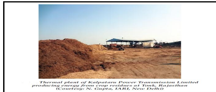
Photo 5 Electricity Generation from Biomass Plant
